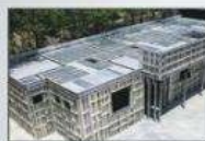
Aluminum Formworks
